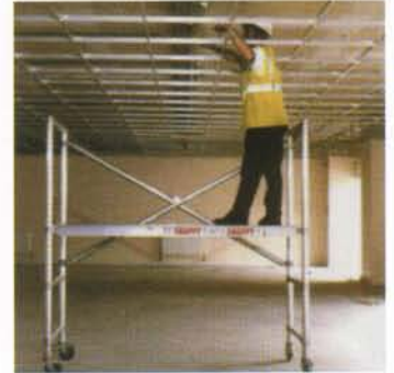
A multipurpose work tool with positive locking swivel castors.
