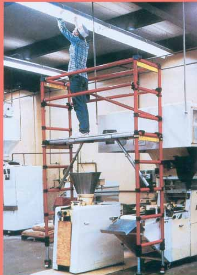
Assembly and maintenance of neon lights
